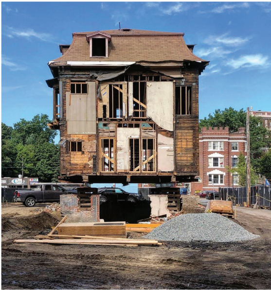
Pictured above and on the opposite page: As part of the Frost Terrace affordable housing project in Cambridge, Mass., the William Frost House was relocated to free up a significant portion of the site for new construction and to communicate the site's residential history along the streetscape.
