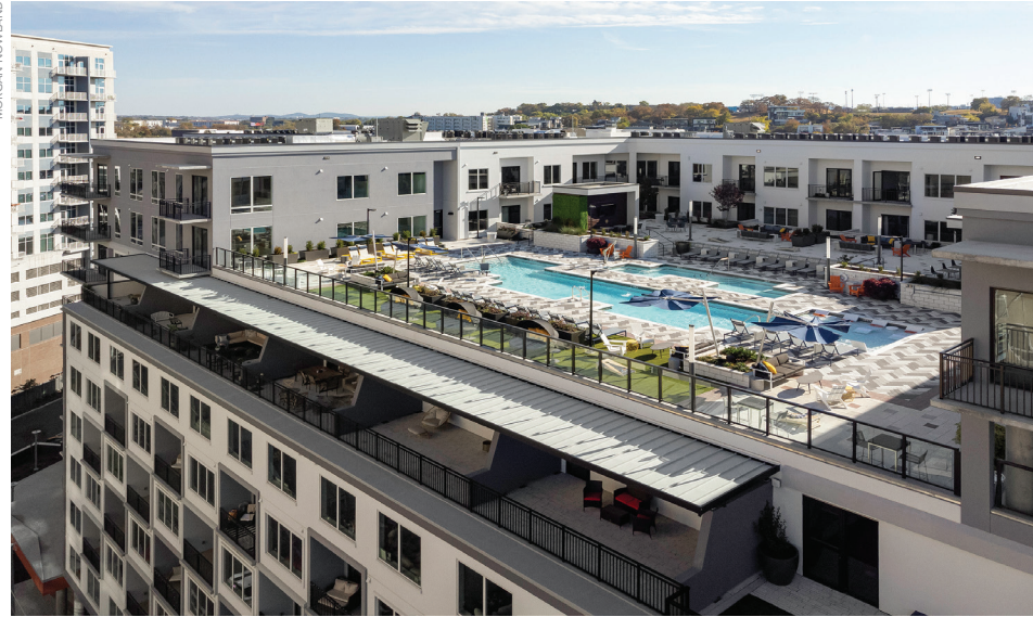
A rooftop pool deck, dog park and spa, bike shop, and large balconies highlight the signature features of the 360-unit, 10-story Aspire Gulch multifamily complex in Nashville, Tenn., designed by Niles Bolton Associates.
