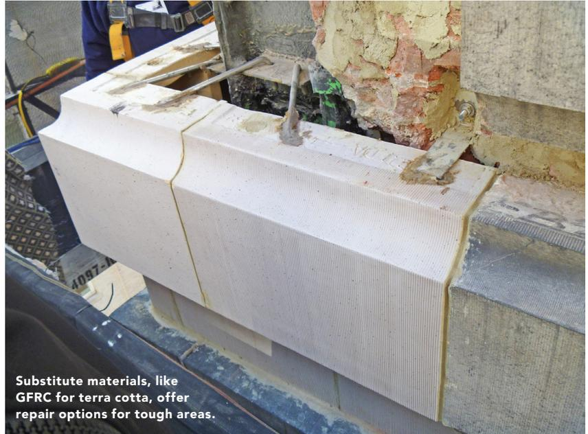
Substitute materials, like GFRP for terra cotta, offer repair options for tough areas.
