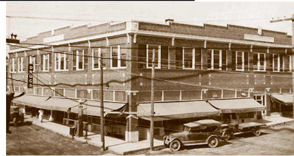
The original Beardmore Block Building in Priest River, Idaho, designed by architect Brian Runberg’s great-grandfather, Charles Beardmore. Runberg learned the history of the building through his grandmother and yearned to reconstruct it to current LEED standards.
