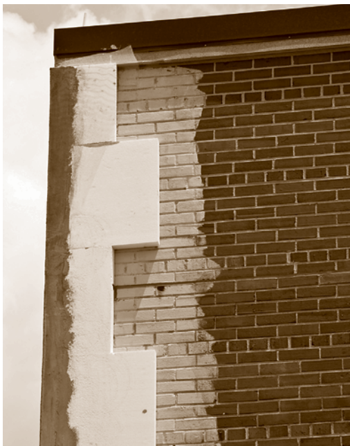
Overcladding in an existing building (left) using an exterior insulation and finish system (EIFS), with the finished work (right). EIFS can be used as overcladding on a masonry wall as long as the masonry is sound, to stop water penetration and improve the insulation R-value of the wall. Insulated metal panels are another increasingly popular overcladding material.
