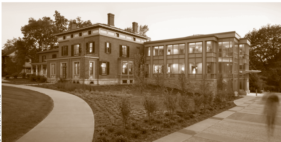
The Welcome & Admissions Center at Roger H. Perry Hall at Champlain College, Burlington, Vt., was certified LEED Platinum in 2011. The renovation and addition to the 150-year-old building restored the historic windows and added interior storm windows to achieve an overall value of R-20 with an air infiltration 60% better than code.
