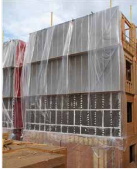
This photo shows how a multi-story wood building can be protected from the elements.
