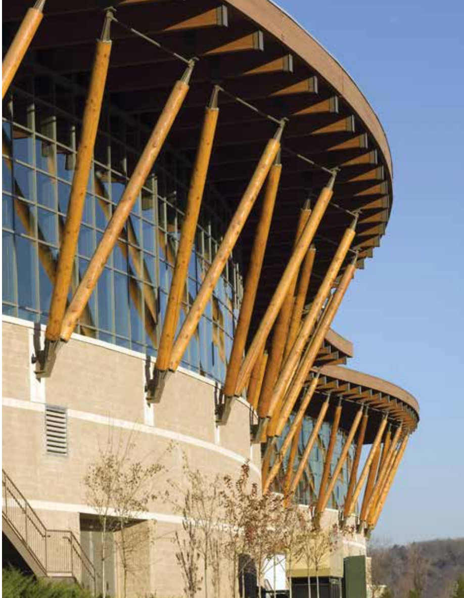
Designed by tvsdesign, the Branson Convention Center in Branson, Missouri, features a large overhanging roof. By sheltering the wood underneath, the roof deflects precipitation and helps to ensure long-term durability.
