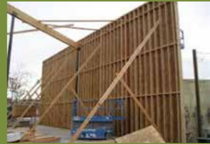
This restaurant in California includes 24-foot walls made from 2-by-8 Douglas-fir.
