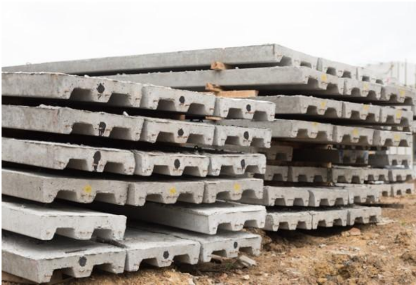
Prestressed Concrete Slabs
