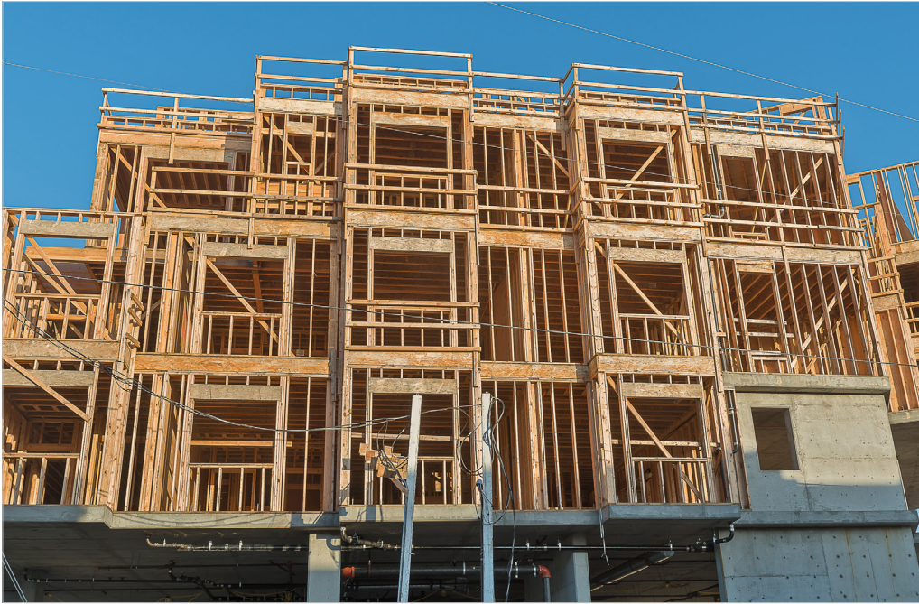
Typical light frame roof and floor systems consist of repetitive framing members such as rafters or trusses with wood structural panel decking. Photo courtesy of Think Wood
