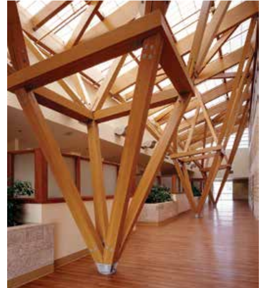
Thunder Bay Regional Health Sciences Center in Ontario, designed by Salter Farrow Pilon Architects Inc., was the first hospital in Canada to gain approval for the use of wood as a primary structural element. Photo by www.naturallywood.com
