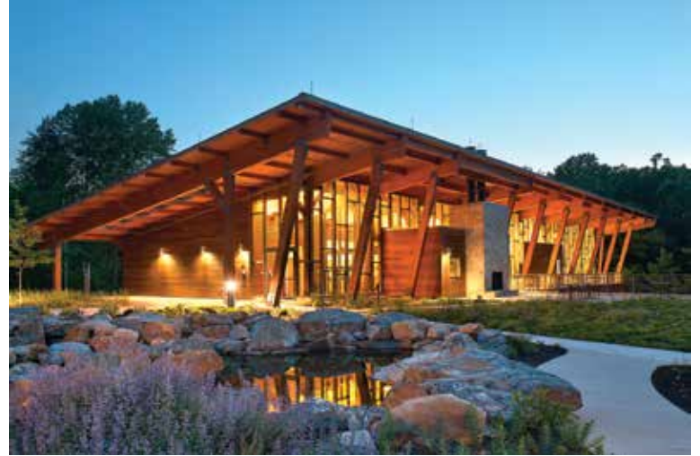
James and Anne Robinson Nature Center; Columbia, Maryland; Architect: GWWO, Inc./Architects; Completed: 2011; WoodWorks Award Winner: Institutional Wood Design. Photo by Robert Creamer Photography and Paul Burk Photography
