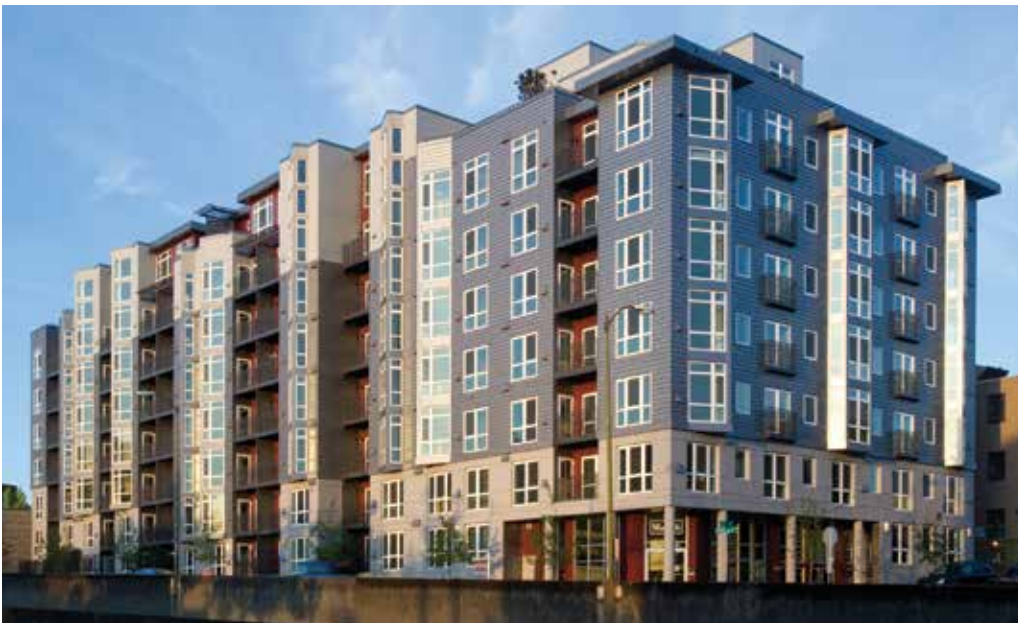
Environmental recognition with local green building programs was a plus for the Marselle Condominiums in Seattle, Washington, designed by PB Architects, but cost was the driving factor in the decision to use wood construction. Photo by Matt Todd, courtesy of WoodWorks
