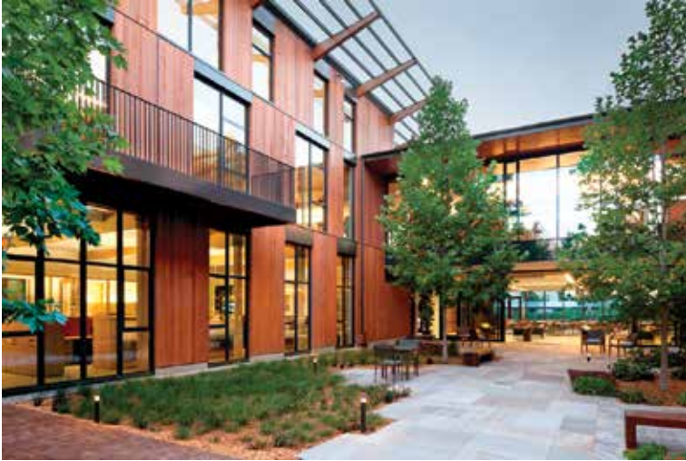
David and Lucile Packard Foundation; Los Altos, California; Architect: EHDD; Completed: 2012; WoodWorks Award Winner: Green Building with Wood. Photo by Jeremy Bittermann; courtesy of EHDD
