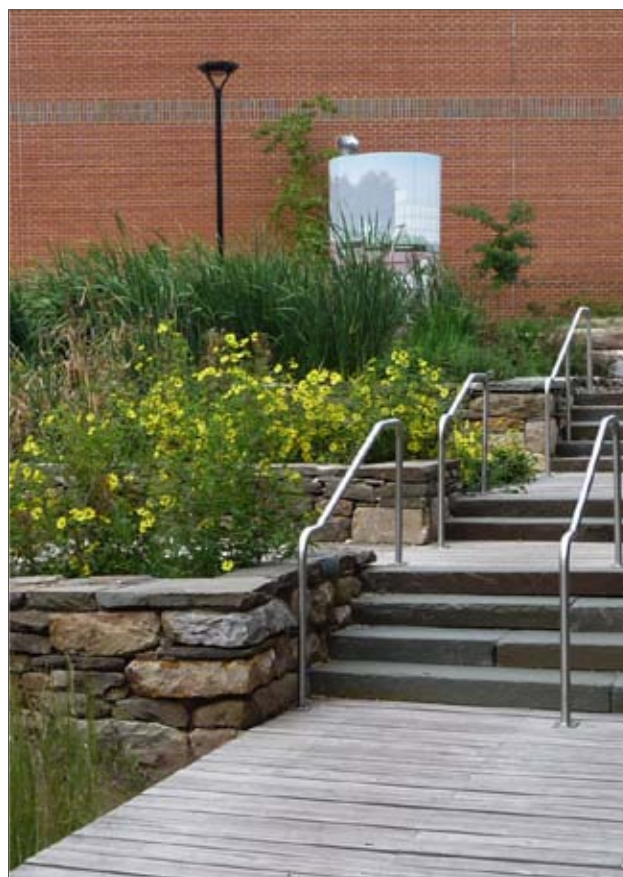
A terraced, subsurface flow constructed wetland designed into the site landscape at Sidwell Friends School.
