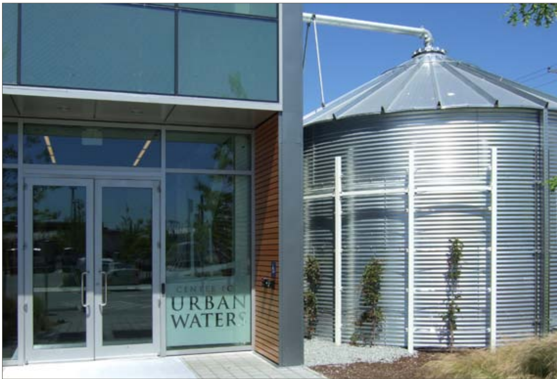
The Center for Urban Waters in Tacoma, WA, harvests rainwater in two 36,000-gallon above ground cisterns.
