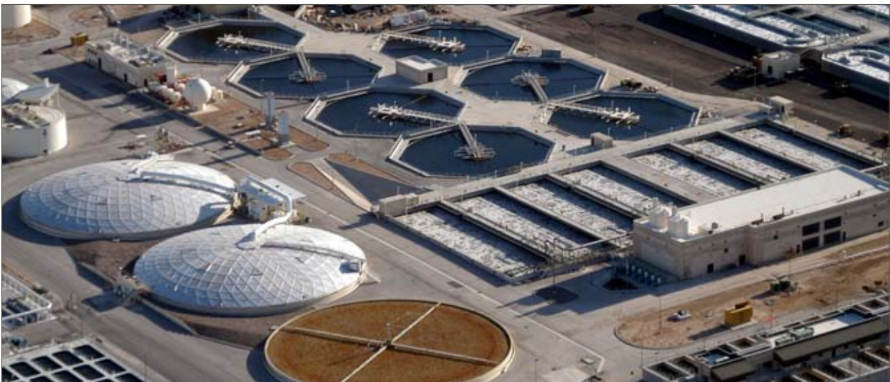
Centralized water treatment facility.
