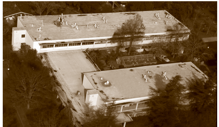
The Sarnafil roofing system that UC Davis chose in 1981 has been protecting critical learning spaces at Robbins Hall for more than three decades.
