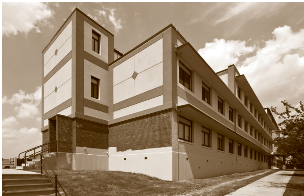
Overcladding in an existing building (left) using an exterior insulation and finish system (EIFS), with the finished work (right). EIFS can be used as overcladding on a masonry wall as long as the masonry is sound, to stop water penetration and improve the insulation R-value of the wall. Insulated metal panels are another increasingly popular overcladding material.
