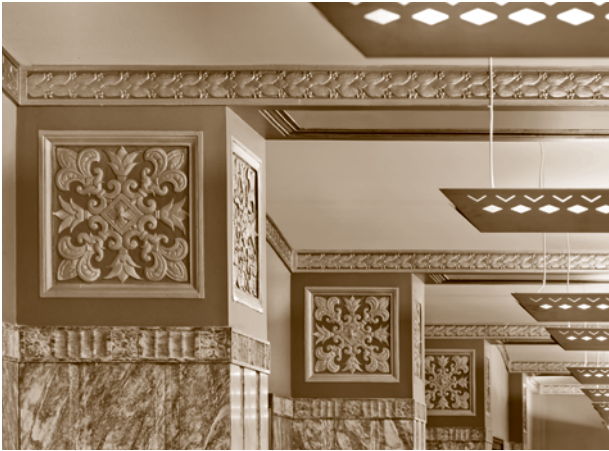
Detail of the intricate restoration work at the John W. McCormack Post Office and Courthouse, in Boston, a 702,000-gsf project completed at a construction cost of $160 million.
