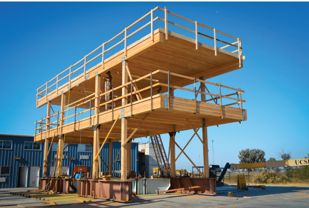
Shake table testing exposes full-scale buildings to simulated seismic events.
