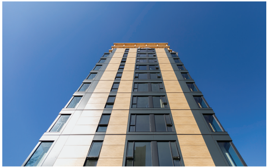
Featuring a hybrid mass-timber system, Brock Commons demonstrates the application of mass timber in high-rise construction.
