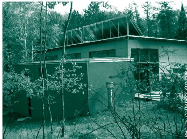
The Waldsee BioHaus Environmental Living Center at Concordia College, Moorhead, Minn., a net-zero energy "Passivhaus" that uses StoTherm NEXt EIFS cladding.
