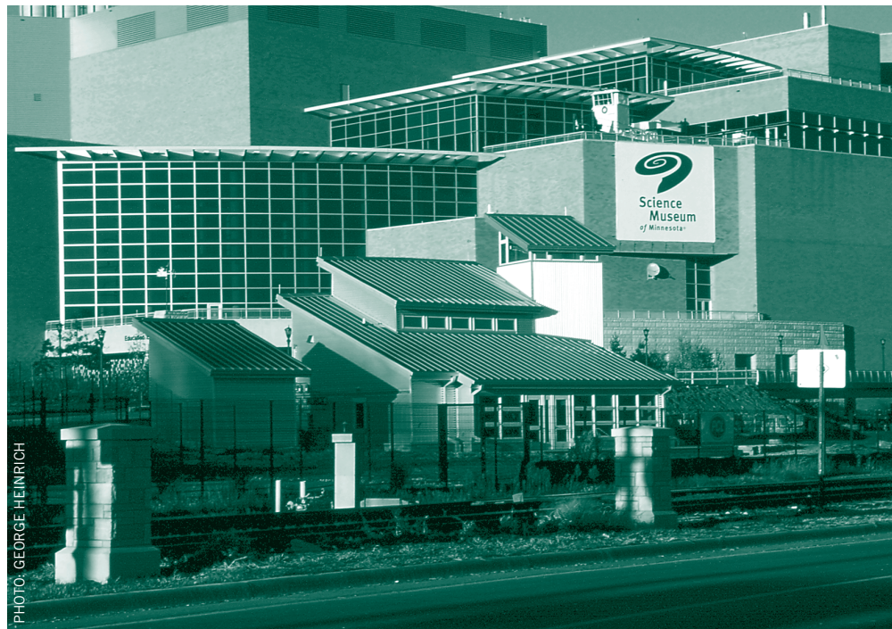
The 1,700-sf Science House (at center in photo) features an 8.8 kW photovoltaic array and ground-source heat pumps. The Building Team consisted of Barbour LaDouceur Design Group (architect), Vareberg Engineering (EE), Martin Mechanical Design (ME), The Weidt Group (environmental consultant), and LS Black Constructors.
